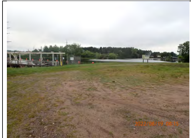
8. View of dam, reservoir, and parking area
