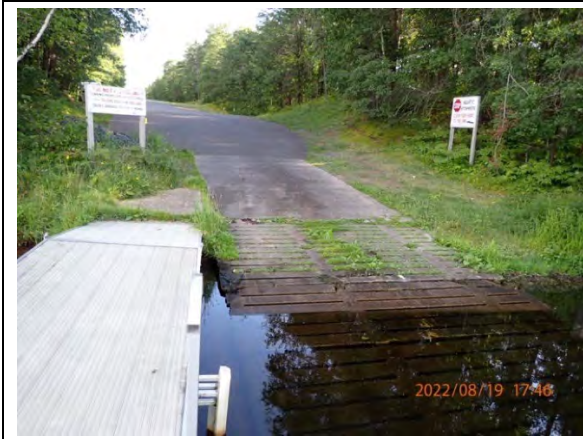
88. Alternate view of boat launch and dock
