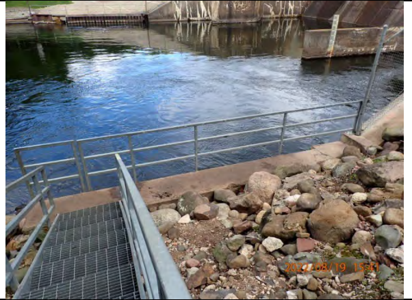
133. South tailwater access stairs and fishing platform
