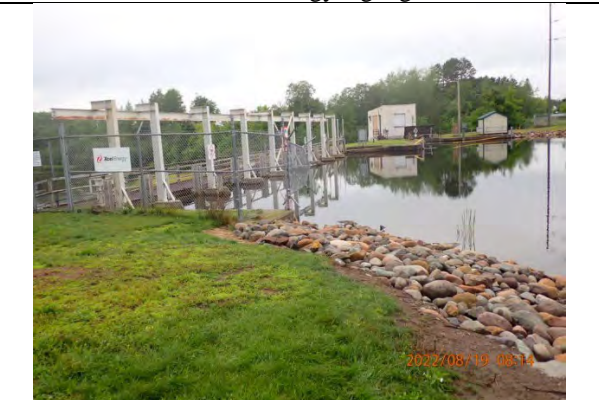
6. Upstream view of dam and reservoir
