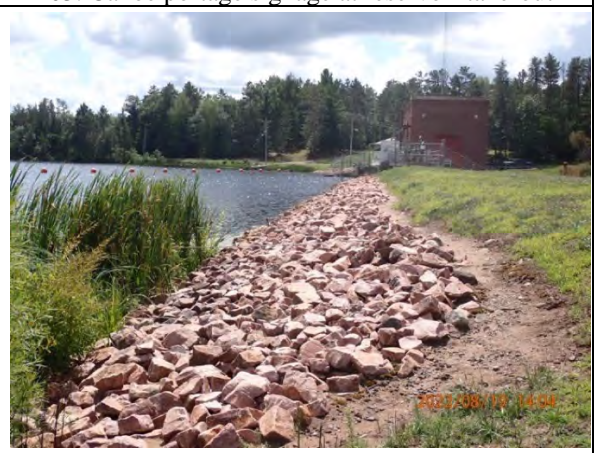
105. View of dam from take-out
