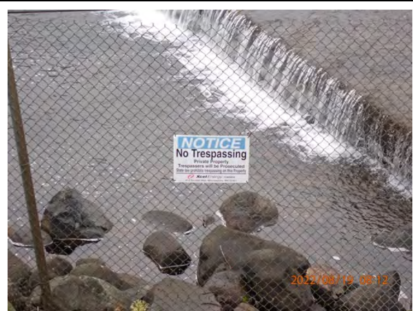
2. Signage downstream of Dam
