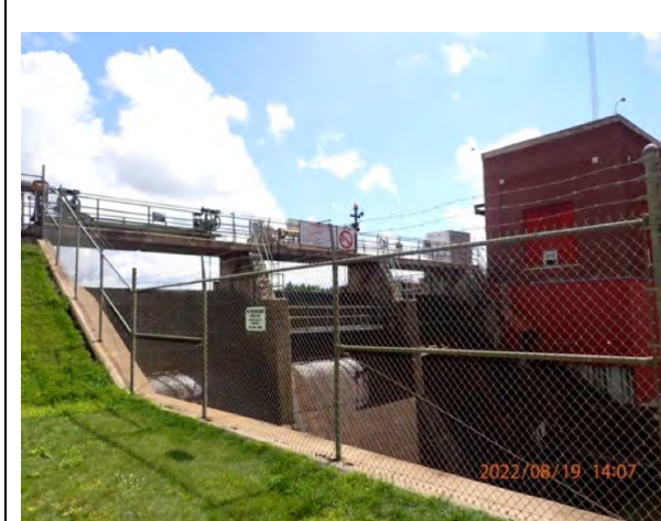
108. Dam and powerhouse
