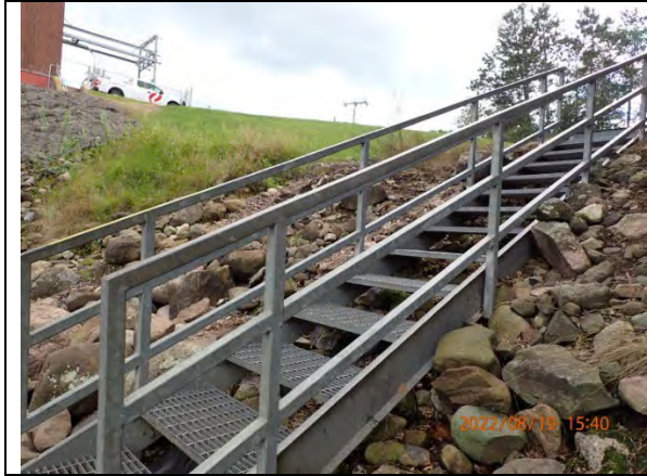
132. South tailwater access stairs
