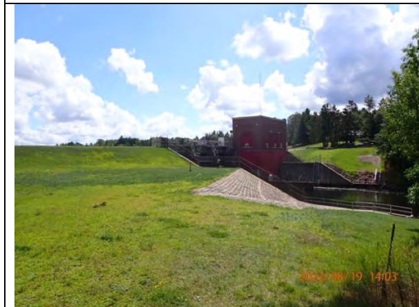
102. View of dam, powerhouse and tailwater
