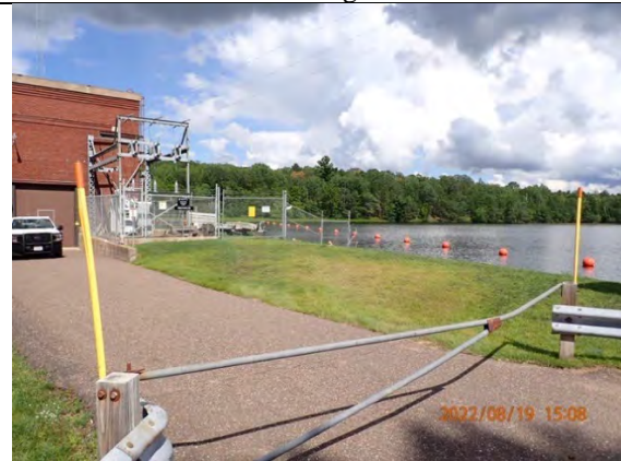
123. Entrance to powerhouse building
