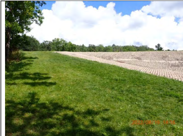
118. View of dam from tailwater fishing area
