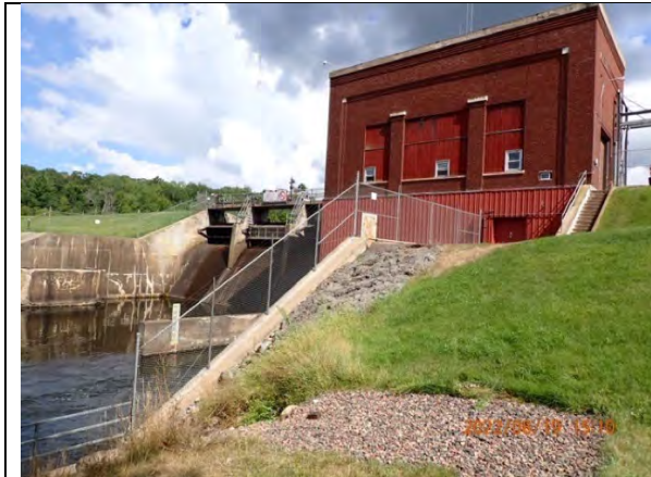
126. Dam and powerhouse
