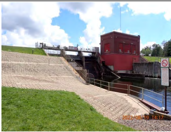
119. View of dam and powerhouse from tailwater fishing area
