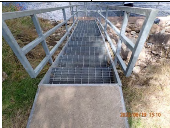
128. Stairs to south tailwater access platform
