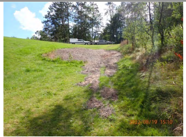
127. View of bank access from tailwater fishing area
