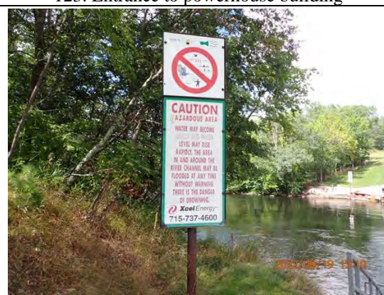
125. Dam safety signage
